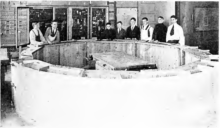
Fig. 41. Silo Form Completed.
